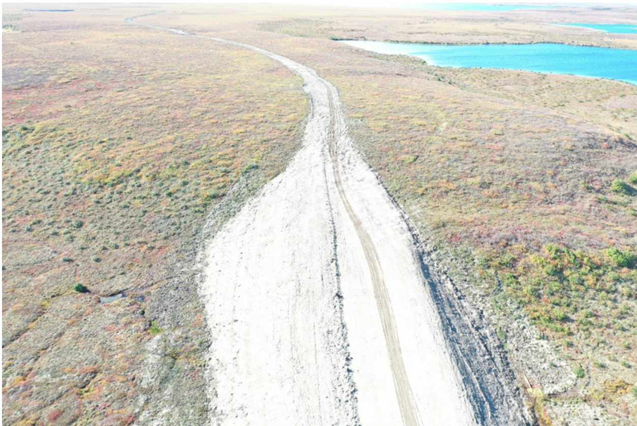
M-18 Access Trail Looking Towards the M-18 Well and Sump – September 2022
